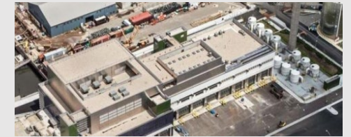
Newtown Creek WWTP
